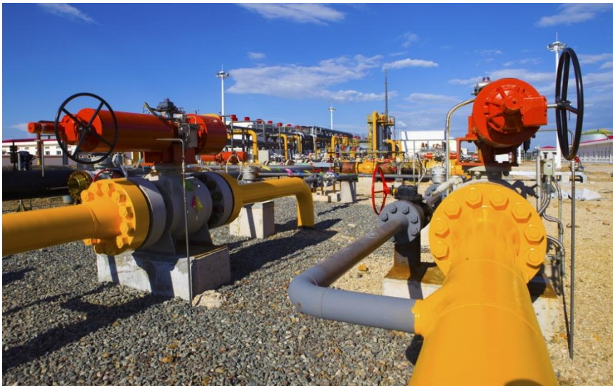
Small Capital Construction
